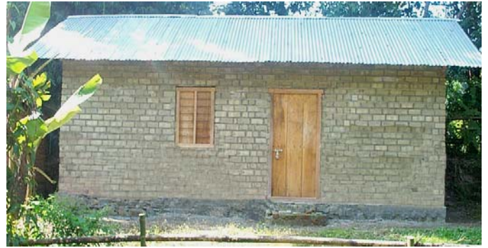
Stabilised Mud Block House for DEWALI, Club
