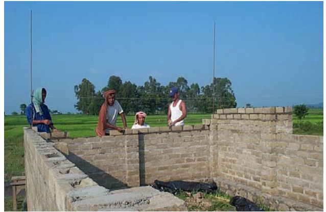
Construction Stage of Mud Block House
