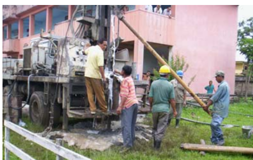
Drilling of tube well at The Govindajee Temple, Imphal.
