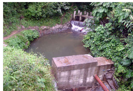
Fore bay tank and diversion weir
