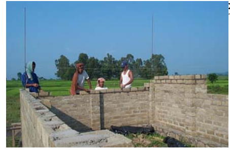
Construction Stage of Mud Block House
