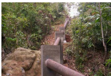
Laid Penstock Pipes with saddle/anchor blocks
