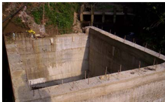
Newly constructed Fore-bay Tank
