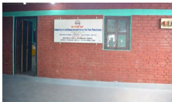
Common facility cum demonstration centre for food processing
