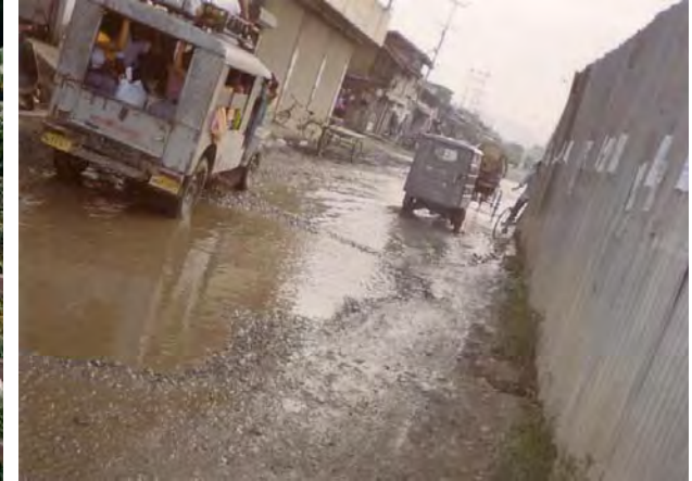
Water-logged road due to poor drainage at Uripok
