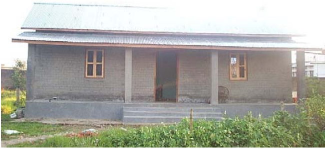
Demo Mud Block House at MASTEC Office Complex
