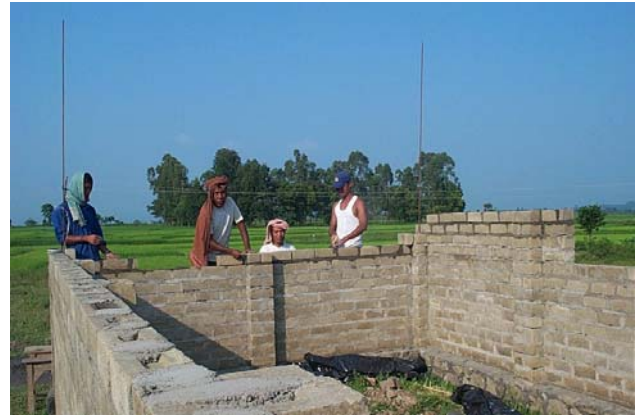
Construction Stage of Mud Block House
