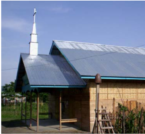
Evangelical Baptist Church ( EBC) before structure was installed
