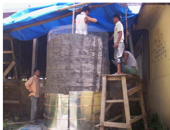
Engineer supervising mason's team during construction period at Govindajee complex
