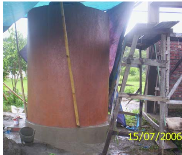
Ferro-cement water storage tank installed at Don Bosco High School
