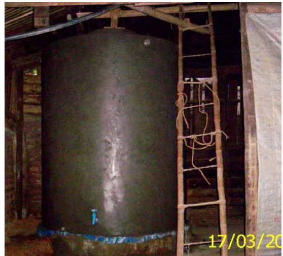
Ferro cement water storage tank at Moreh, bordering Myanmar
