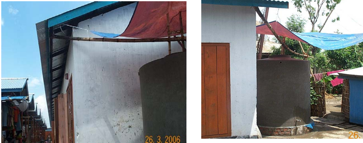
Ferro-cement water storage tank for Thoubal district under curing period
