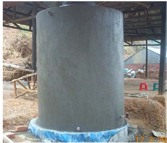
Ferro-cement tank at Langol
