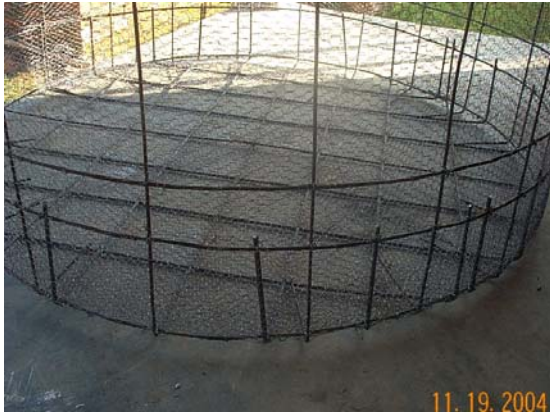
Skeletal of bottom portion of the tank
