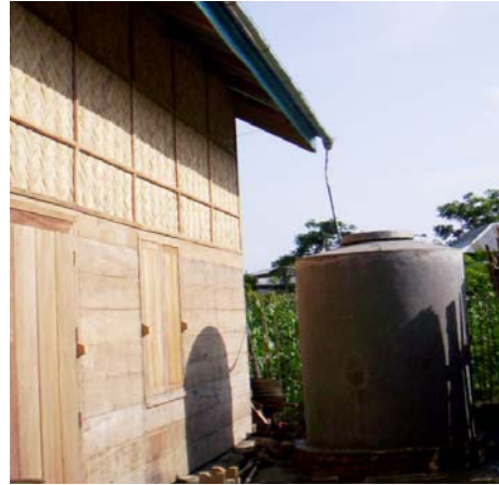
E. Baptist Church with roof top rain water harvesting structure. Elemveng.
