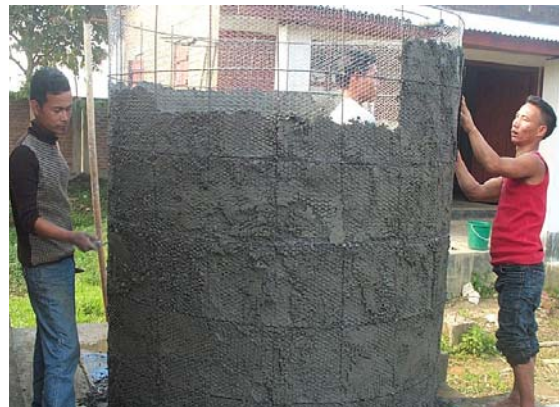
Plastering inside wall of the skeletal body
