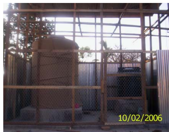
Ferro-cement Water Storage tank at Wangkhei, Imphal East Dist
