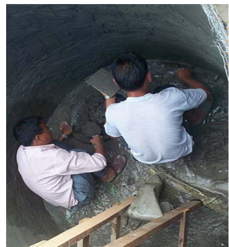
Plastering bottom floor of the tank (inside)
