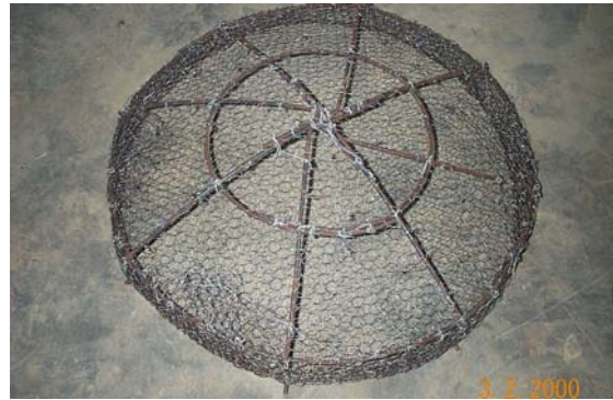
Roof man hole cover ( skeletal)
