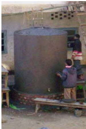
Structure at Motbung
