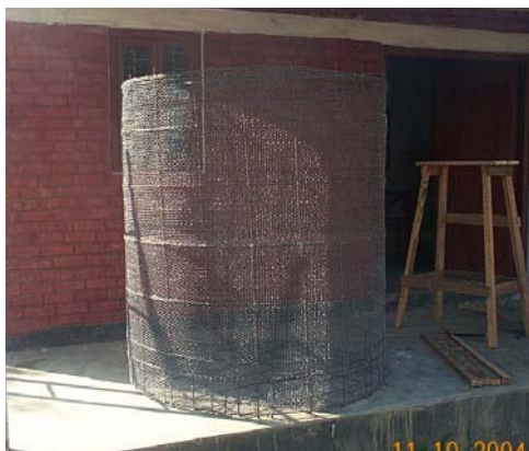
Skeletal of tank tied with wire mesh
