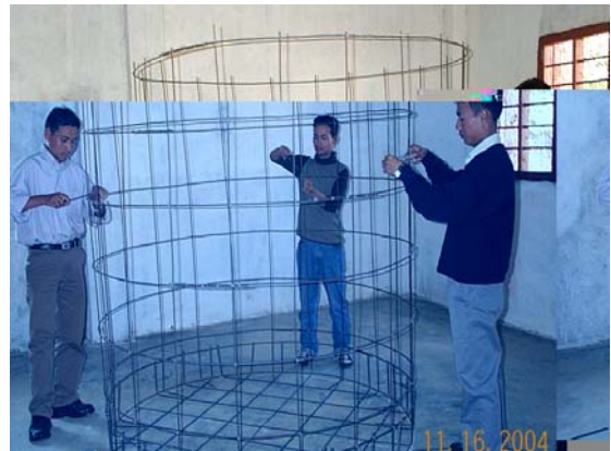
Fabrication of skeletal cage of tank
