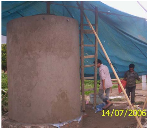
Ferro-cement water storage tank installed at Don Bosco High School
