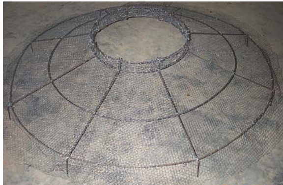
Roof cover with man hole (skeletal)
