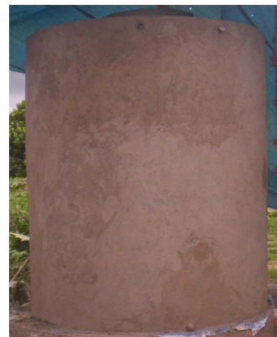
Ferro-cement tank installed at Moirang in Bishnupur
